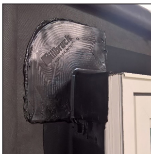
Fig 1: ME241 EPDM Corner, shown bonded after ME220 VV application (bond with OT015)
